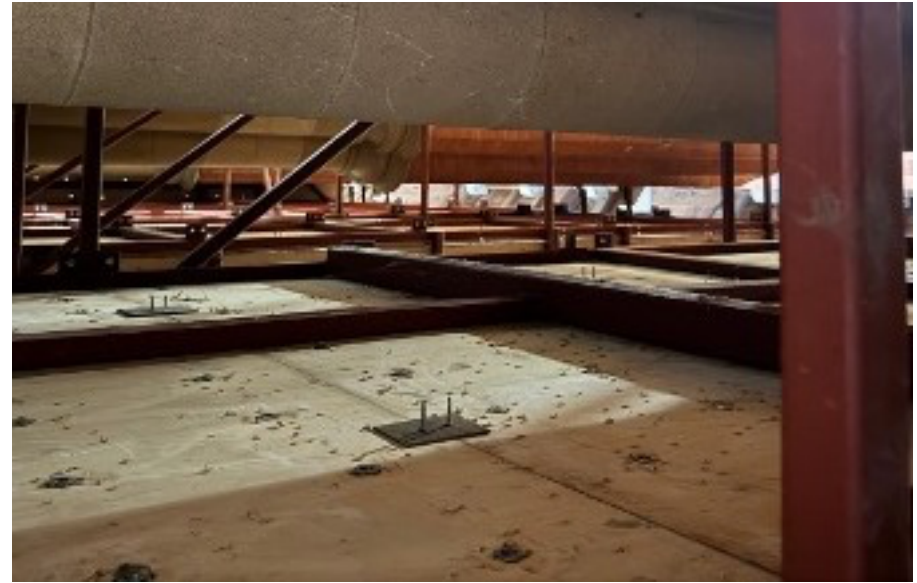
P06 Reverse face of the climbing installation beside a historic arcade column, showing the red-painted steel sub-frame, plywood backing, protruding bolts and connection components. The frame is to be dismantled without levering or bearing against the column.
