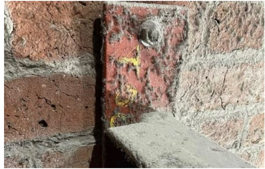
P06b Close view of a steel member, end plate and fixing into historic brickwork. The fixing position, hole and adjacent mortar joints are to be recorded before compatible repair is agreed.
