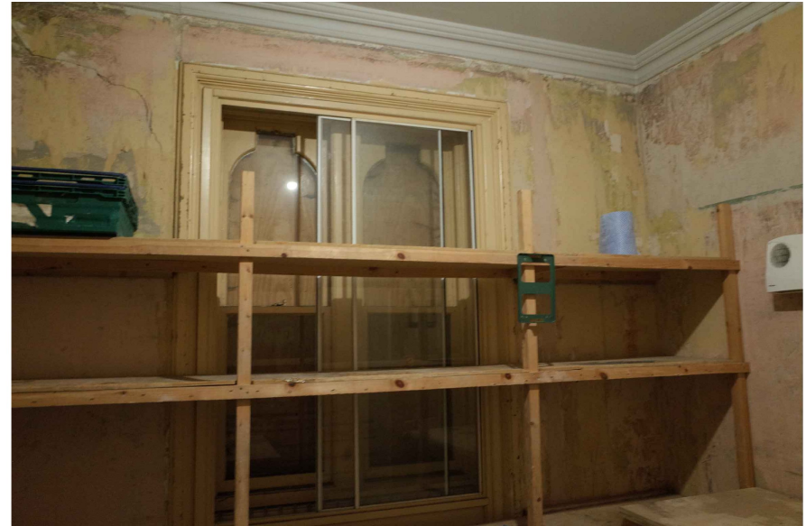
V05b Complete existing north-wall view, including the window opening, cornice and later shelving within the room.
