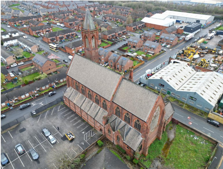
P01 Daytime aerial view of the whole church, including the tower, Nave and aisle roofscape, principal elevations and surrounding townscape.
