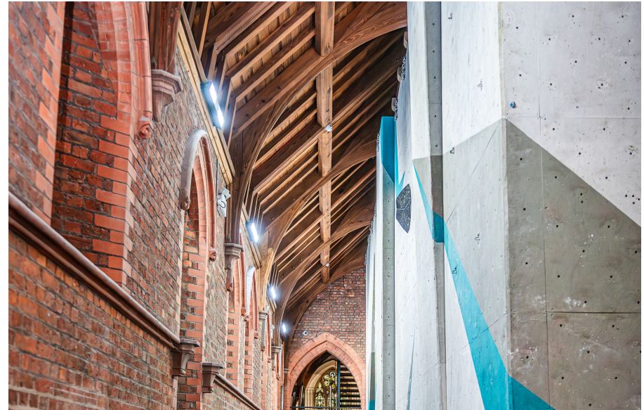
P04 North Aisle looking west. The retained brick wall, roof and floor remain legible beside the climbing structure; the new level doorway is formed farther east as detailed by BTP.
