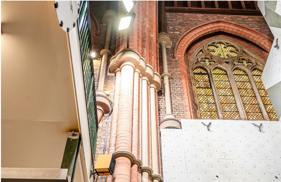
P05 Climbing wall immediately beside historic brick arcading, stone dressings and roof structure. Protection and controlled removal are required throughout.
