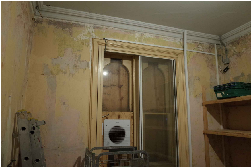
V05a Complete existing west-wall view, including the window opening, cornice and surrounding finishes to be retained behind the independent lining.
