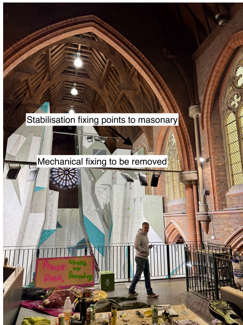
Figure 4 — High-level stabilisation fixing interface
