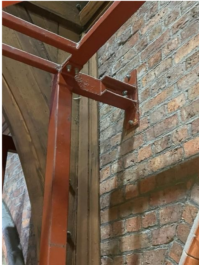
Figure 5 — Representative steel wall plate fixed to historic masonry
