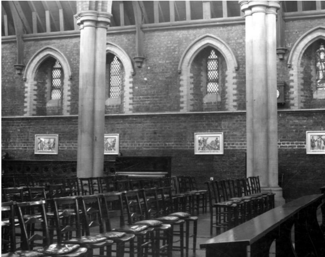
Figure 9: Interior of the Church in 1969 – north aisle. (Source: Manchester Central Library GB127.m70240)
