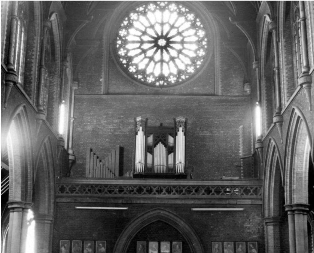
Figure 7: Interior of the Church in 1969 – west end.
